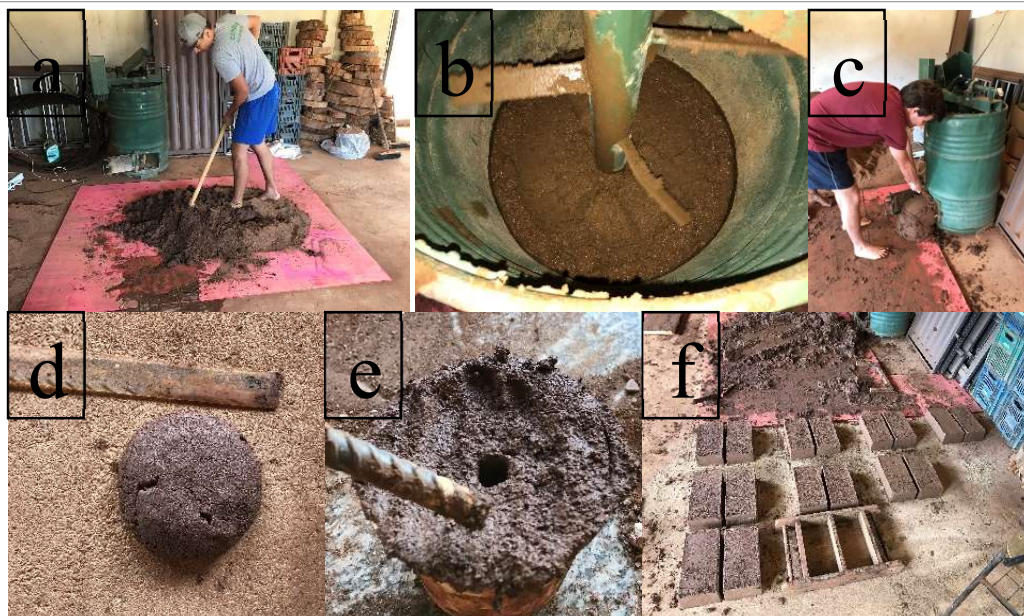
FIGURE 4. Production steps and humidity tests.
