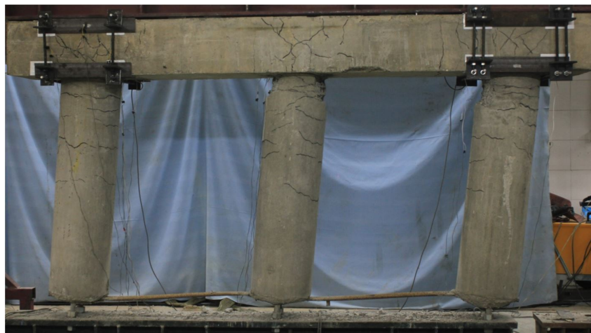
Figure 13: Damage modes of specimen B, Fracture of the longitudinal bars of the middle column, complete failure of plastic hinge, bar slippage of the longitudinal bars of the external columns and failure in cap beam of the left connection at relative displacement of 5.6.
