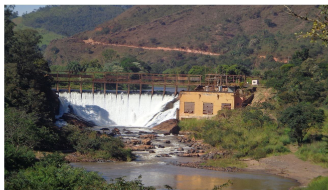
Figure 2. View of the downstream of the Salto do Paraopeba SHP.
